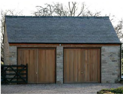
Typical Image: Courtyard and adjoining garage
